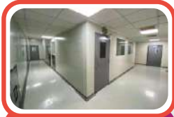
Epoxy Flooring Areas
